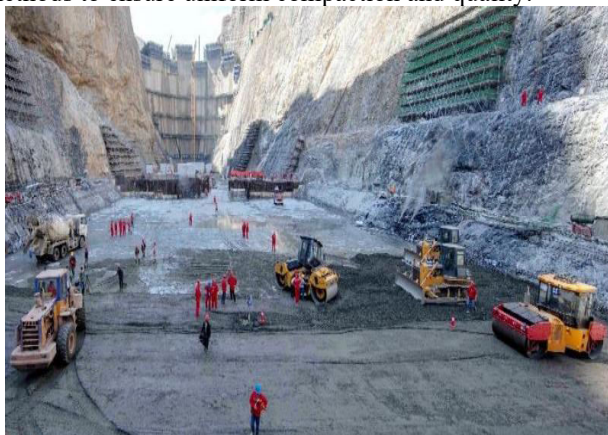
Figure 2: Smart Compaction Concrete Dam Construction
