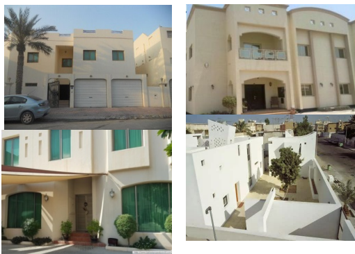
Figure 1: A typical villa in Juffair Area with its fence and surrounding open space (Source: the author)..
